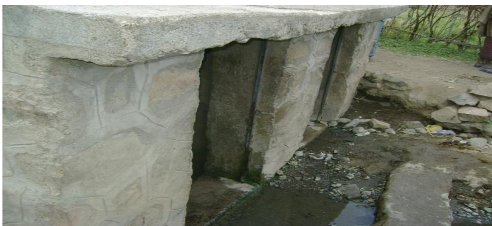
Figure 4: Chachatu Hot Spring Water Rooms
